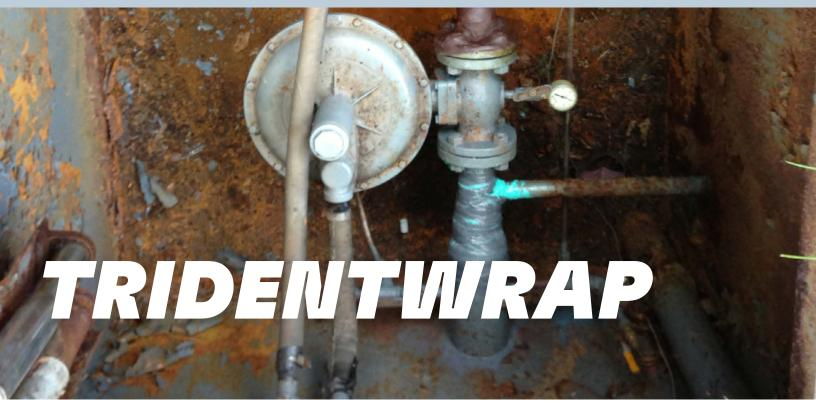
TridentWrap Riser Reinforcement Kits repair non-leaking natural gas risers, enabling you to repair corroded piping without shutdown or riser replacement. The TridentWrap System is prepackaged in diameter-specific kits to eliminate atmospheric corrosion, provide mechanical strength, and restore the pipe to its original integrity.
