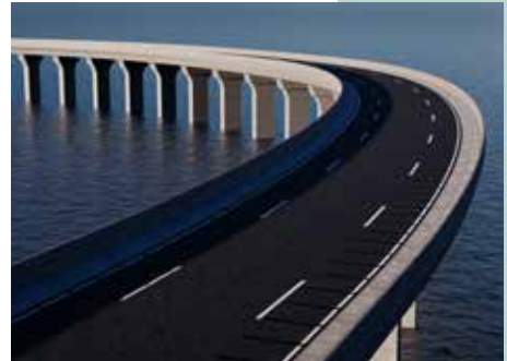
NSM Bar Bridge Strengthening
