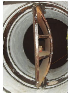
Steel substrate prepped for application
