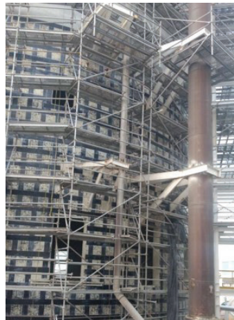
Scaffolding and Installation of LOCTITE FRP System
