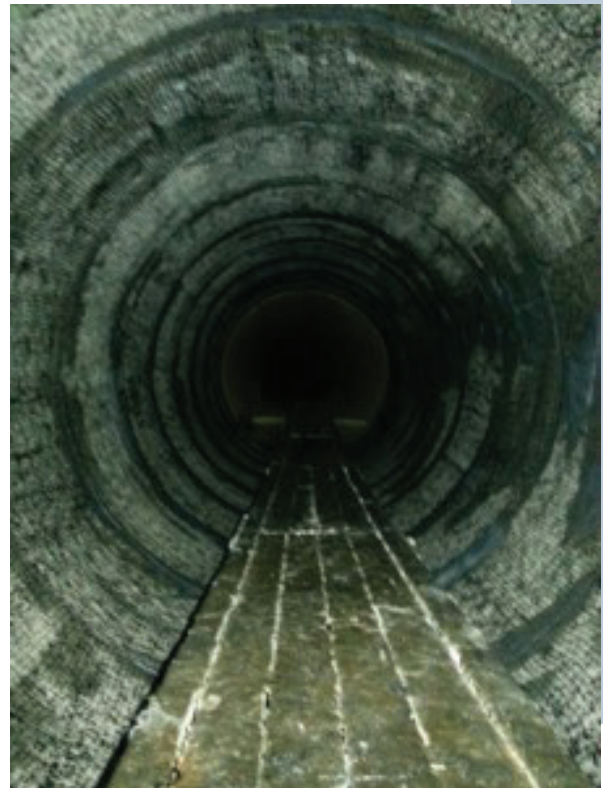
Eagle River Station penstock after rehabilitation with LOCTITE FRP System
