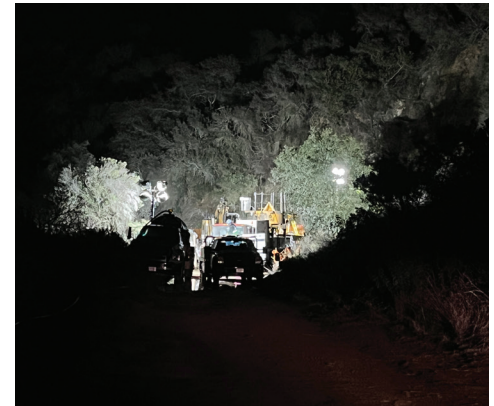
External job site
