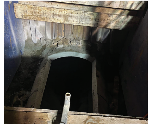
Pipe access point
