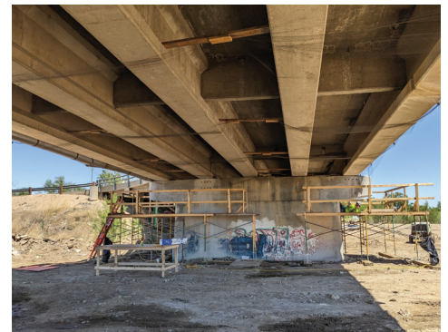
Scaffolding in place to enable pier access.
