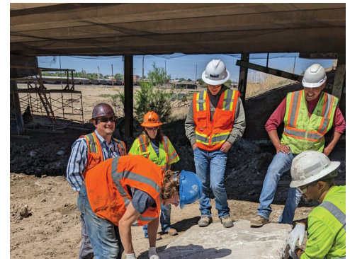
Onsite training taking place.
