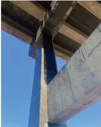
Completed application of RenewWrap FRP.
