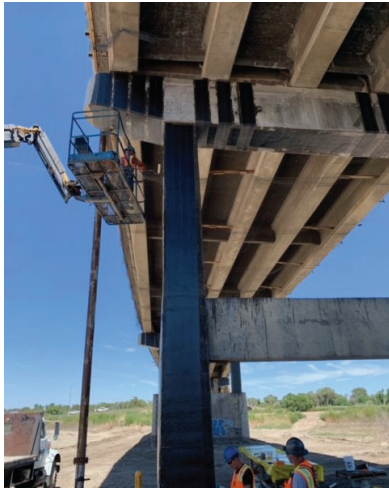
Cherry picker used to apply FRP at height.
