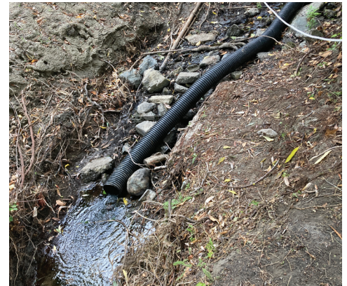
Discharge of bypass outside culvert
