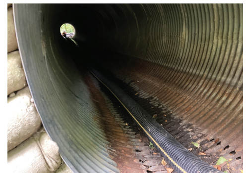
Bypass through culvert to be rehabilitated
