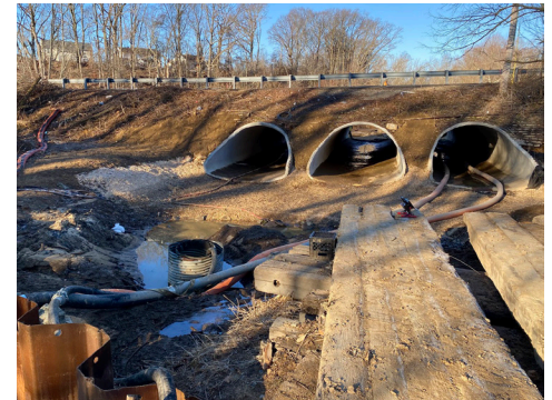
Bypass in Place
