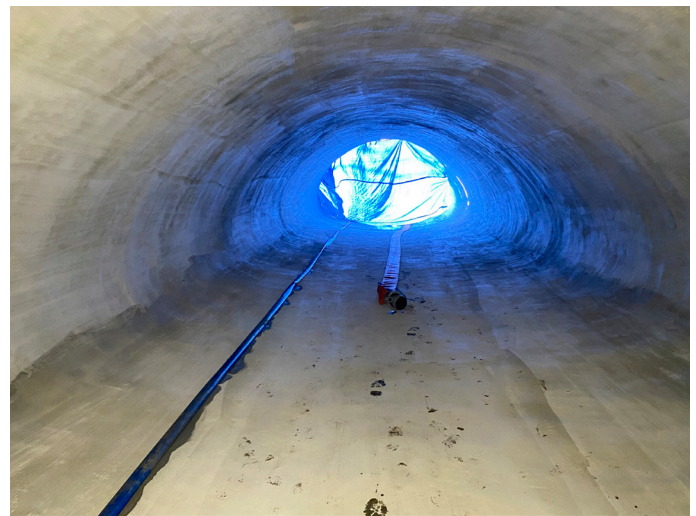
Completed geopolymer application
