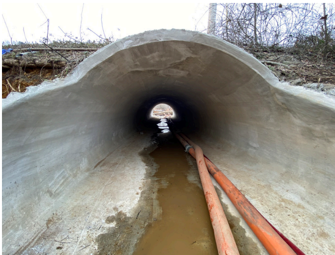
Completed application, bypass still in place
