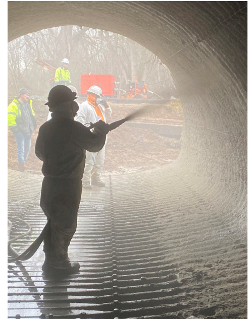
Shotcrete application of geopolymer liner
