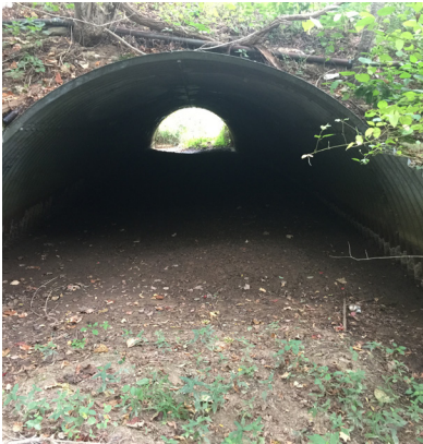
Deteriorated Culverts
