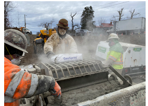
GeoSpray being prepared
