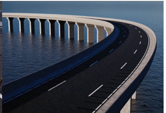
NSM Bar Bridge Strengthening
