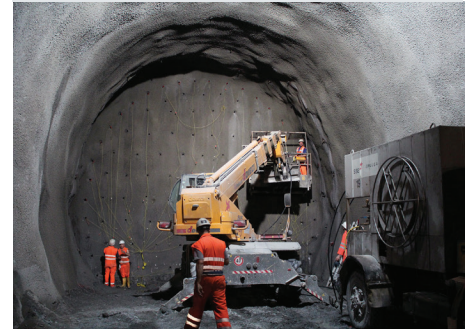
GeoRoc - designed for the surface reinforcement and weathering protection of soils, rock and coal strata.
