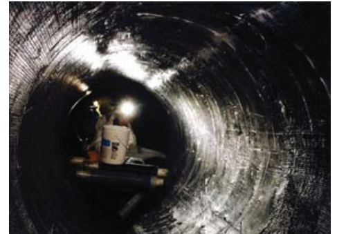
Hand application of Tyfo® Fibrwrap®
