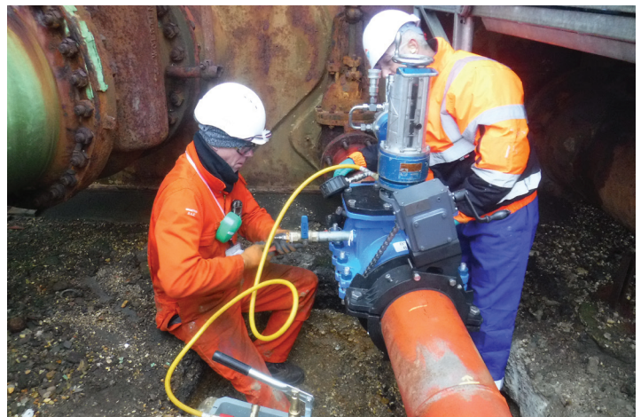
EM Machine fit and pressure test taking place
