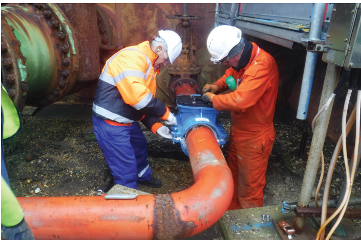
Valve body installed ready for EM machine to be fit
