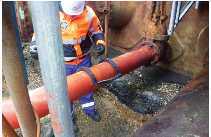
Pipe marked up ready to take EZ Valve
