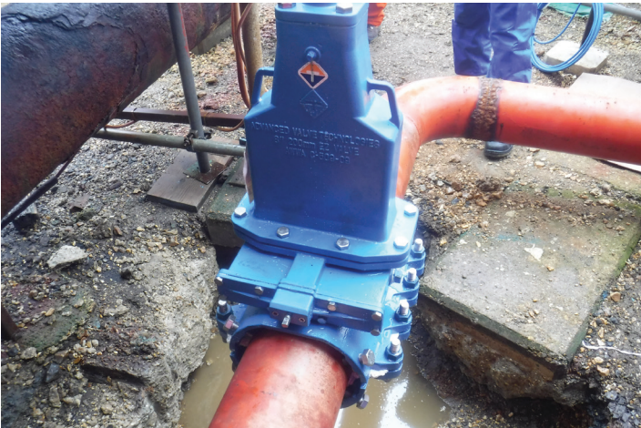
Completed install of AVT EZ Valve
