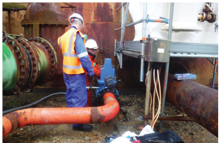
Bonnet installed awaiting gear box removal
