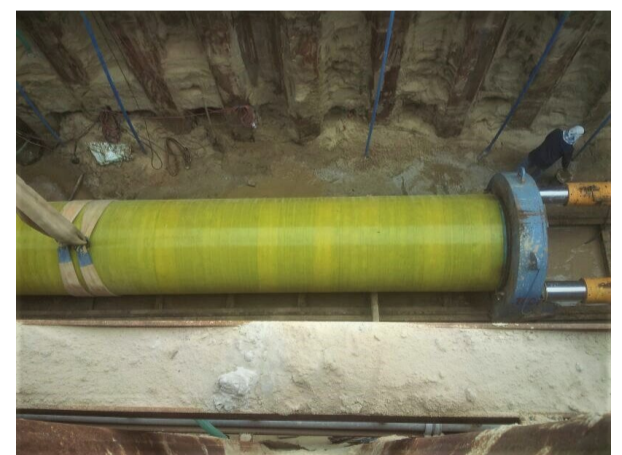
The abrasion-resistant fiberglass composite coating protects the pipe from mechanical stresses and scarring.
