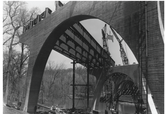
Arch Pier During Construction, circa 1964
