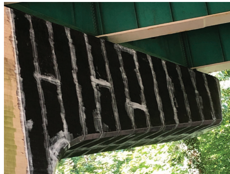
Completed Cantilever Wrap on Arch Pier
