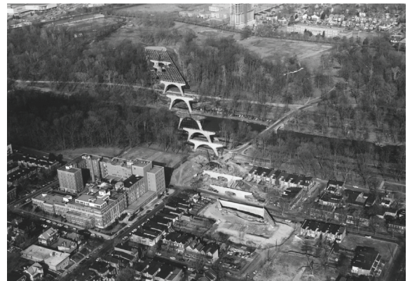
Aerial View of Bridge Piers Prior to Superstructure Installation, Jan. 30, 1964
