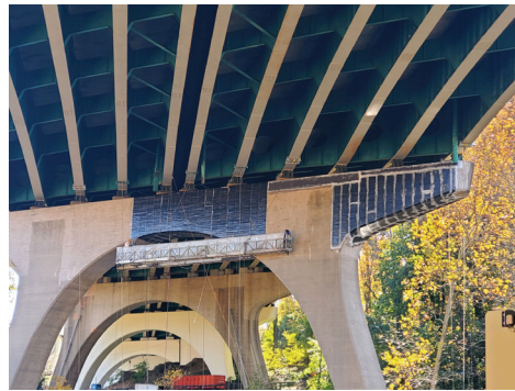
40’-0” Swing Stage at Pier 6
