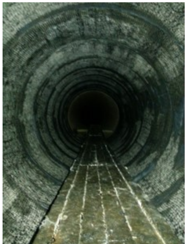
Eagle River Station penstock after rehabilitation with Tyfo FRP System
