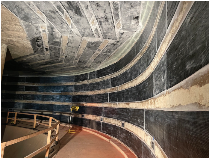
Reservoir partial plan, showing Tyfo SCH-41-2X for seismic reinforcement of the concrete walls and slab diaphragm, and Tyfo BC at the wall-slab joints.
