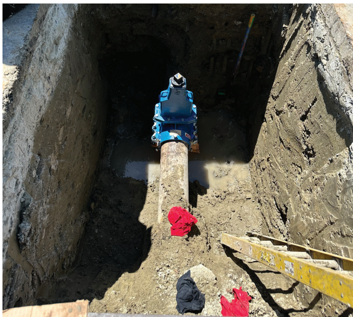
AVT EZ Valve installation complete with bonnet in place
