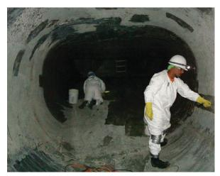
The general requirements of the American Concrete Institute's 440.2R-08 guide were followed for flexural strengthening with additional limit states investigated, such as CFRP debonding, steel reinforcement yielding and concrete crushing.
