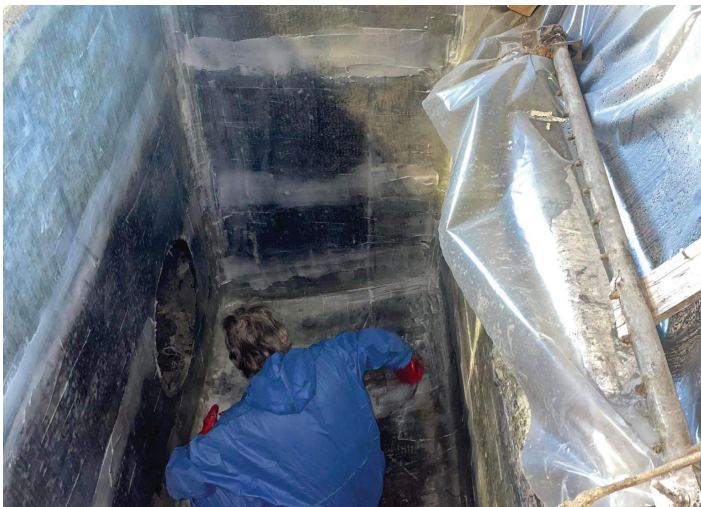
Application of Tyfo system
