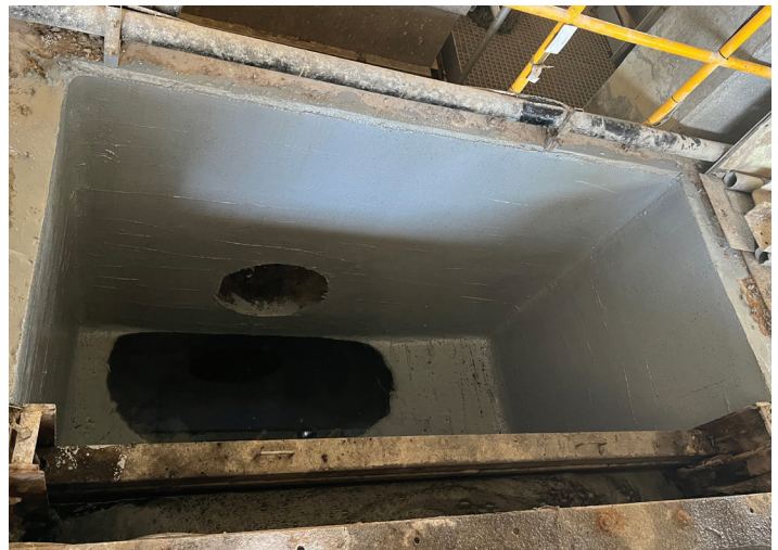
Completed rehabilitation of tank
