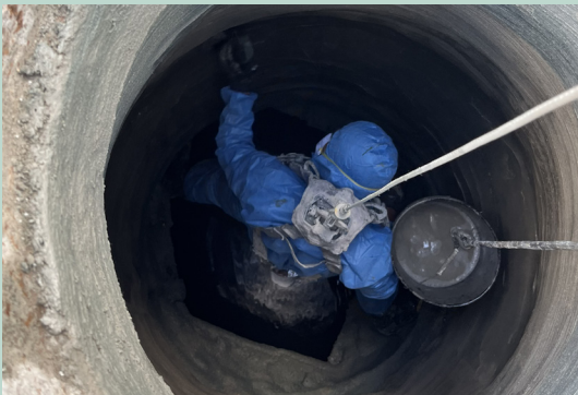
Installation in progress
