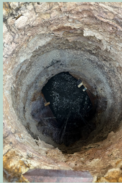
Severely deteriorated manholes
