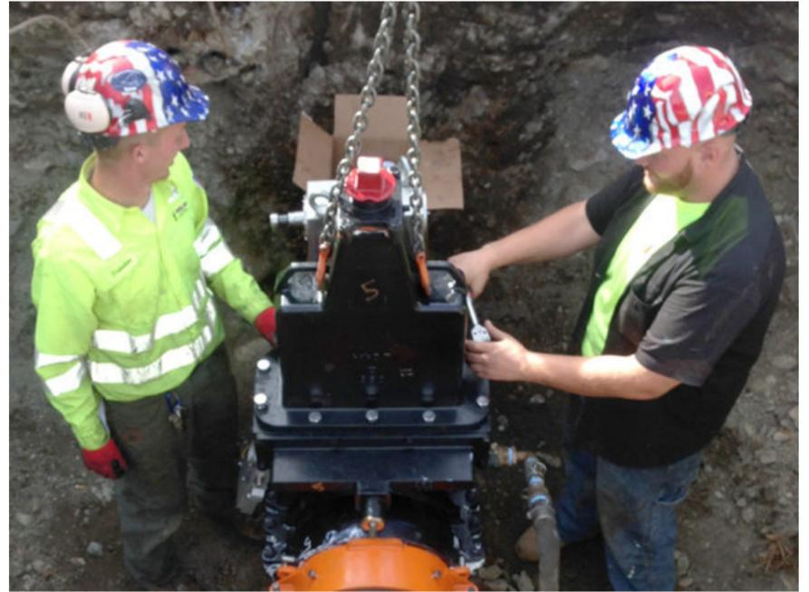
The successful installation of the two valves on this line brought the number of Hydra Tech's AVT EZ Valve™ repairs to 537 in less than 5 years.
