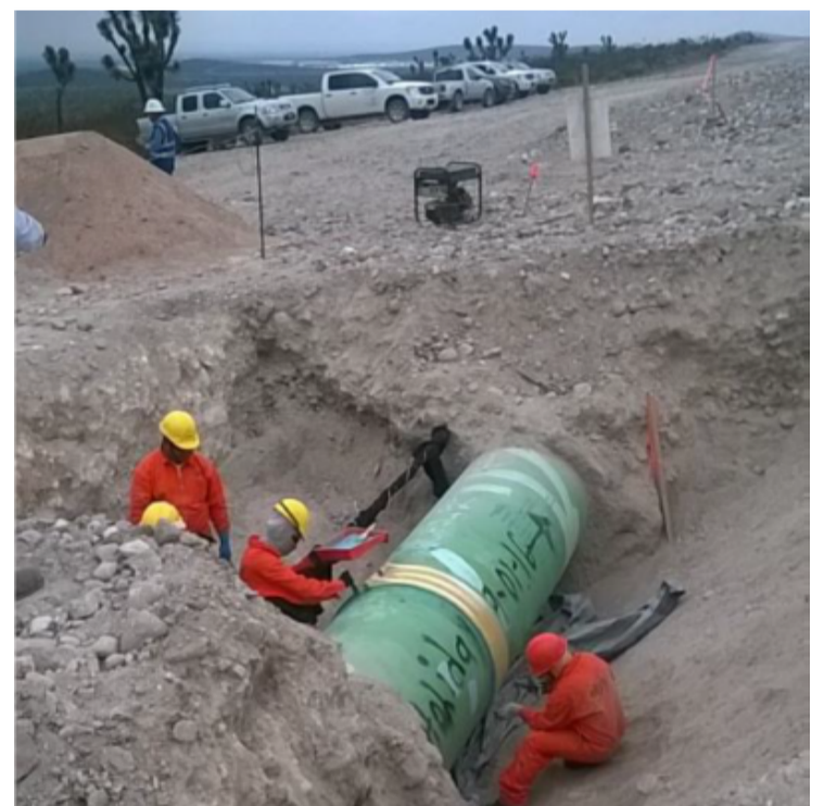
Composite Sleeve Repair
