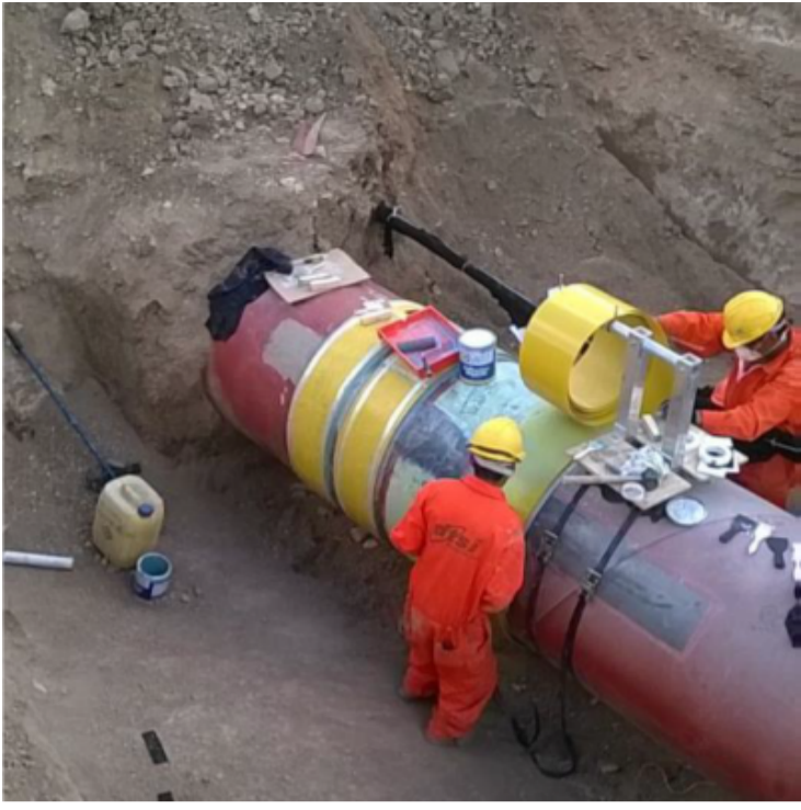
Composite Sleeve Repair
