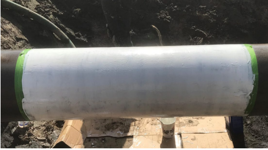
Installers applied a special two-part epoxy coating to the repair zone.
