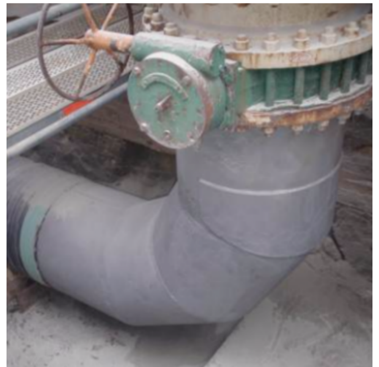
Area to be repaired after sand blasting
