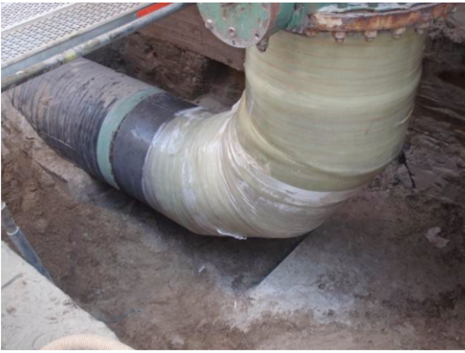
First 4 layers installed and left to cure
