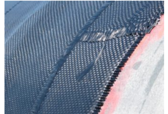
Each successive layer of DiamondWrap® increases the pressure rating.
