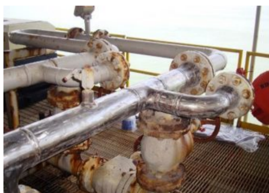
The repair area is cleaned to SSPC.SP11 surface preparation standards.
