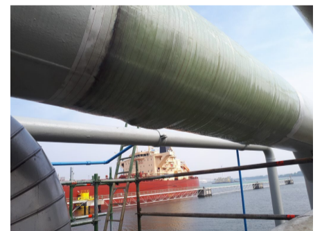
Lower Side of Repair
