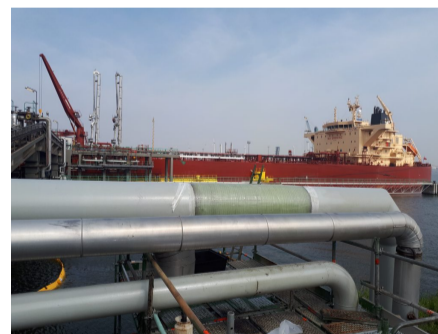
Repair in context
