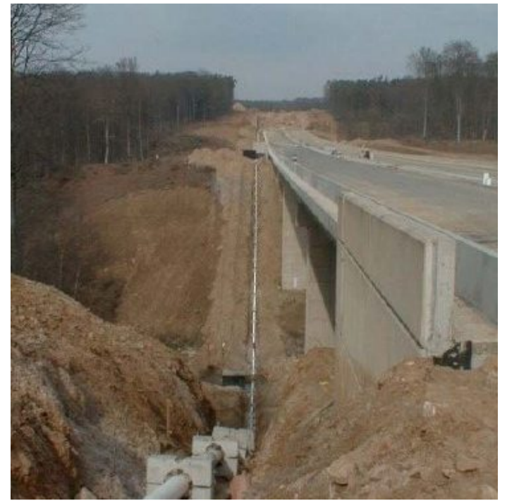
Pipeline coated and pipe support construction completed
