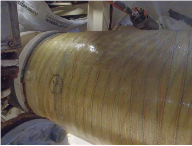
Leaks in the original repair had to be addressed before the CSNRI solution could be installed.
