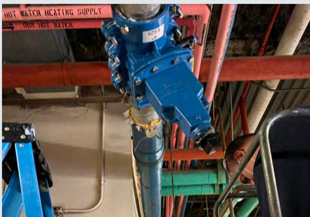
End rings and gear box removed, restraining bolts tightened, valve install complete
