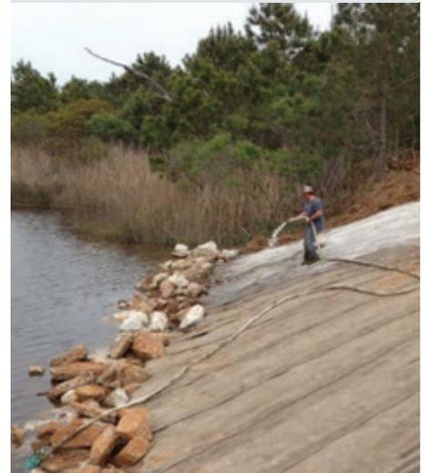
Concrete Cloth GCCM installed and hydrated on slope.
