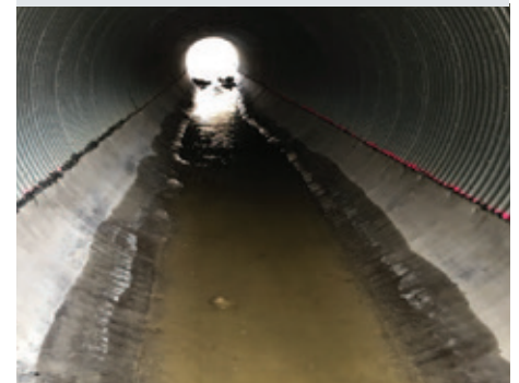
Rehabilitated culvert invert with CC8.
