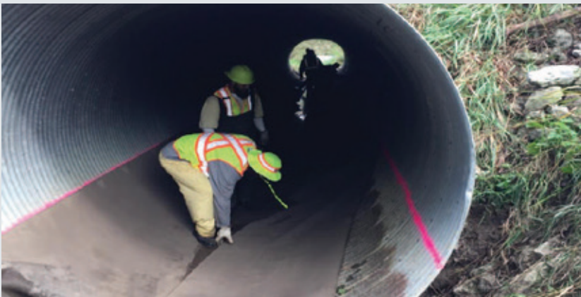
Laying CC8 sections longitudinally in invert.
