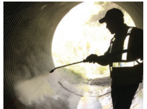
Hydrating CC8 to harden fabric.
