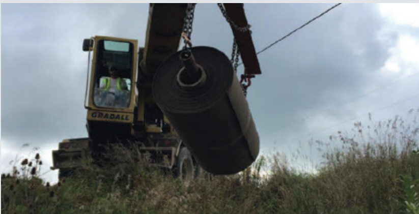
CC8 fabric roll lowered into culvert.
