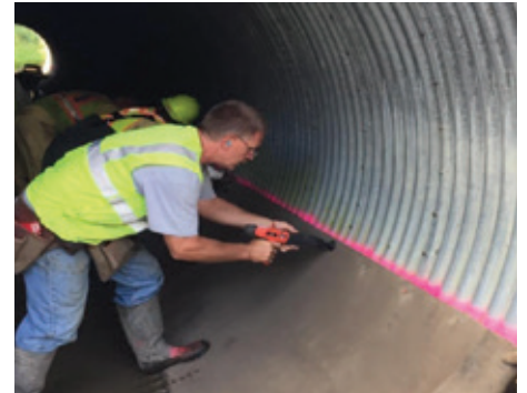
Securing CC8 with stainless steel screws.
