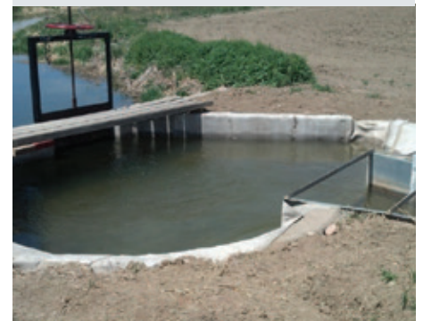
Filled irrigation collection and distribution structure after repair.
