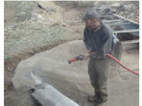
Hydration of repair site.
