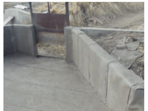
Repair site fully lined with Concrete Cloth GCCM.
