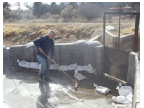
Brooming site to hydrate material.
