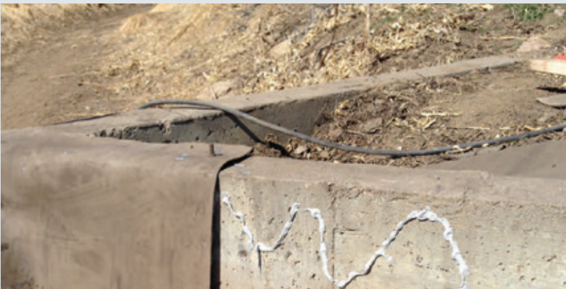
Adhesive applied to vertical wall for separate GCCM panels.
