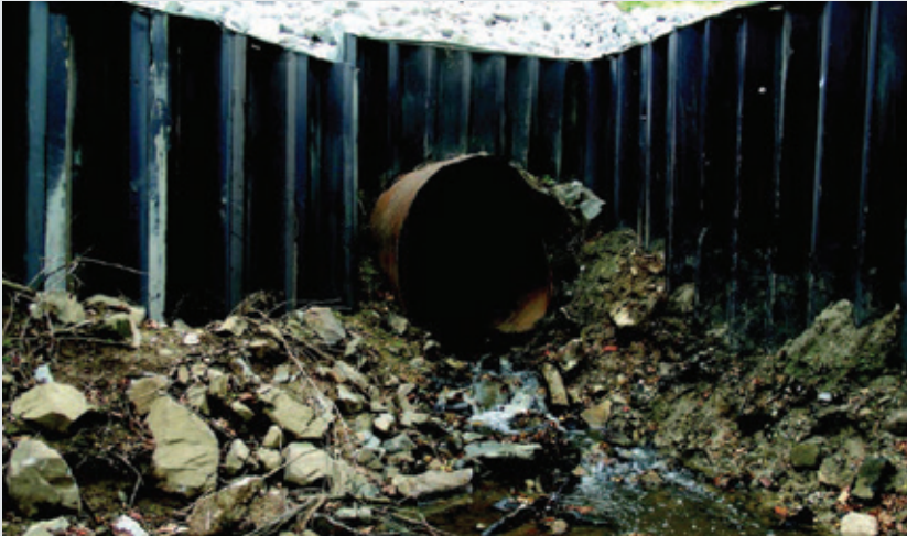
Head wall of pipe on river outfall.
