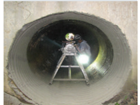
Starting of the GeoSpray Lining.
