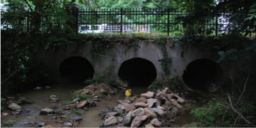
Inlet view of the 3 CMP Culverts to be lined.
