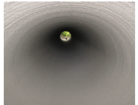
The completed 1" GeoSpray mortar lining.
