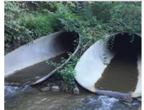
Twin culverts in use after GeoSpray mortar rehabilitation.
