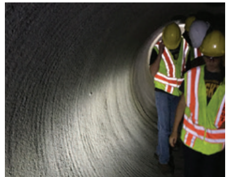
Inspection of lining by MDOT bridge personnel.
