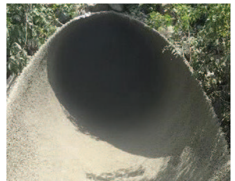
Completed geopolymer lining.
