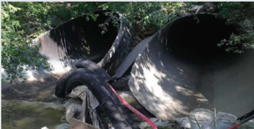
Installation of diversion pumping system.
