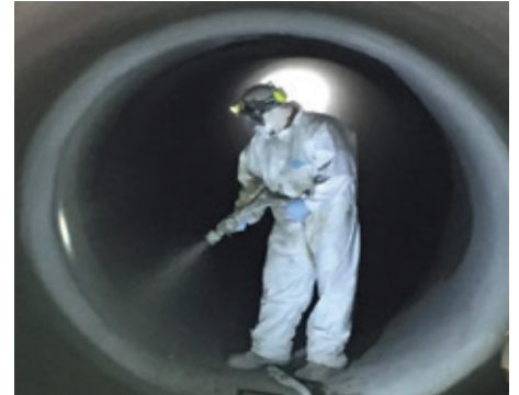
Hand spraying placement of geopolymer lining.
