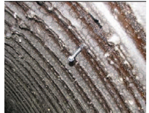
Gauge screws were set for thickness measurement of the liner.
