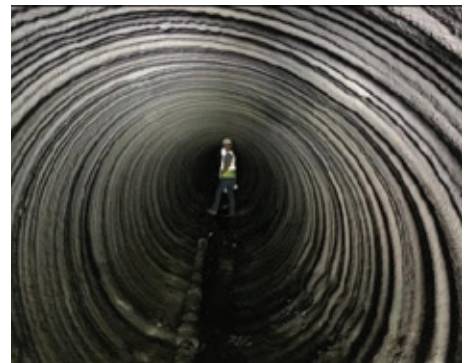
Inspecting the pipe after the second pass of GeoSpray mortar.
