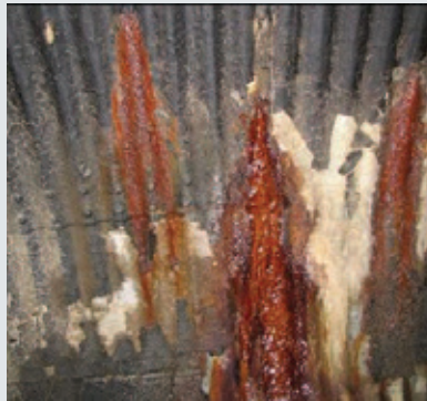
The pipe had severe infiltration, some ovality and a previous asphalt coating.
