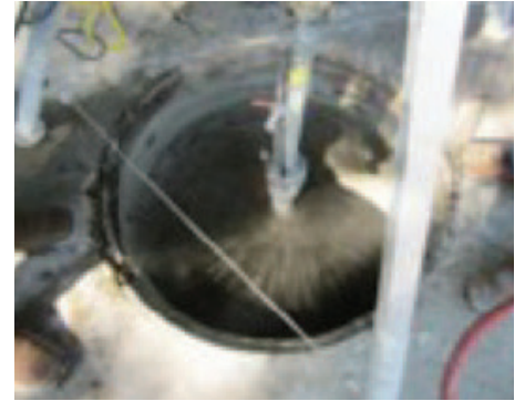
Centrifugal spraying of GeoSpray geopolymer.
