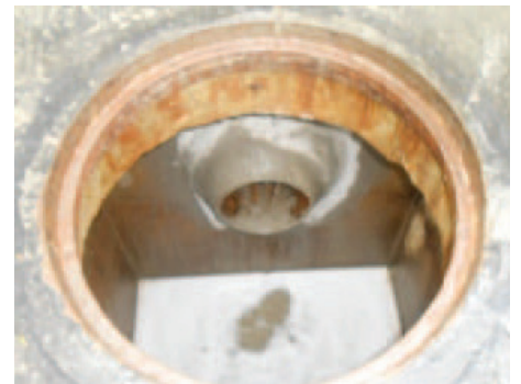
One of several hundred leaching and deteriorated manholes.
