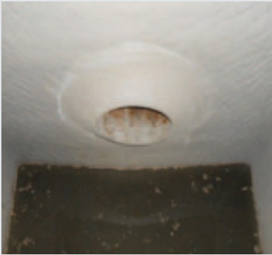
Manhole renewed with GeoSpray geopolymer.
