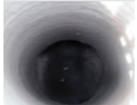
Completed manhole ready for service after eight hours.
