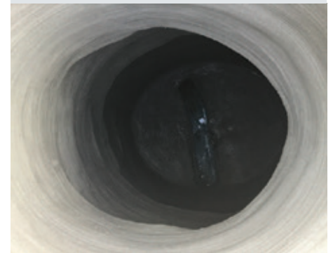
Completed manhole rehabilitation.
