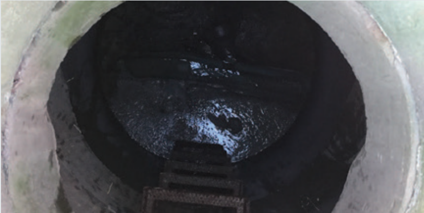
Concrete manhole prior to rehabilitation.
