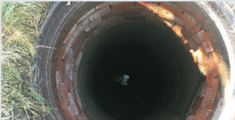
Brick manhole prior to rehabilitation.
