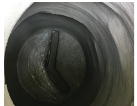
Completed manhole rehabilitation.
