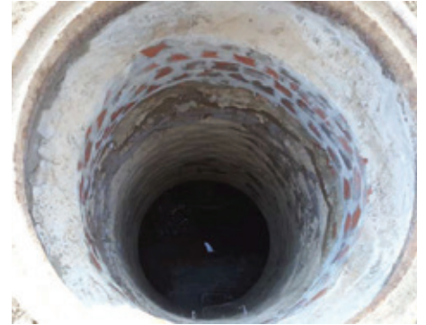
Manhole prior to spraying.
