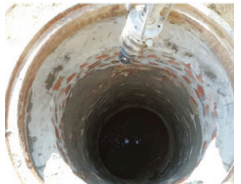
Start of GeoSpray mortar application.
