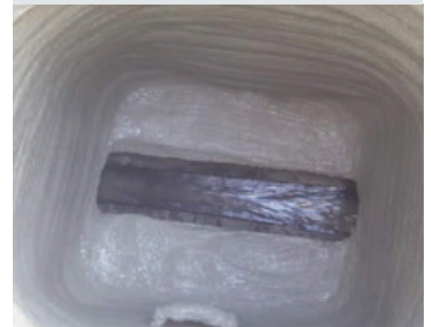
Like-new manhole and bench after GeoSpray mortar application.
