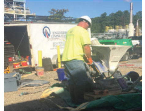
Equipment set up for manhole repair.
