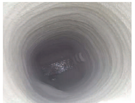
Completed manhole repair.
