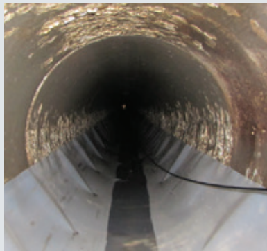
36" folded liner pulled in place.
