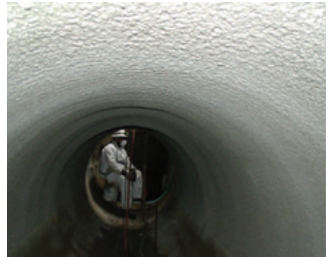
In the process of the lining application
