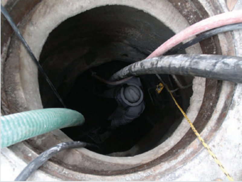
The complete GeoSpray lining system fits through a standard manhole with no excavation needed.
