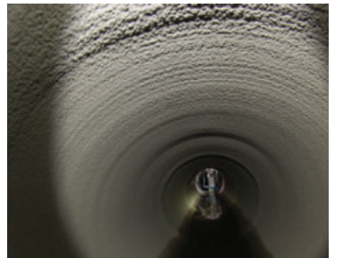
Completed GeoSpray mortar liner.
