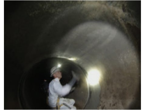
Applying GeoSpray mortar to joints that are infiltrating.
