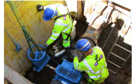
EM (end milling) machine removed and bonnet ready to be mounted
